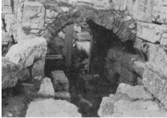
The Heridanos stream converted into a sewer at Ceramicos (photo from Papademos, 1975)
