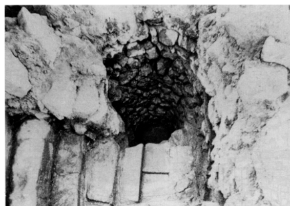
Well-spring located in the eastern wing of the Zakros Palace (Platon, 1974)
